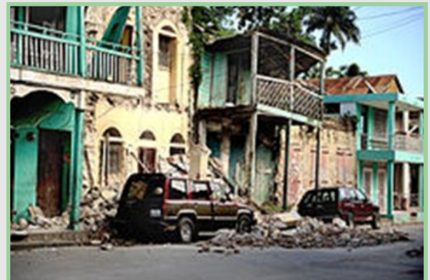
Damaged buildings in Jacmel
