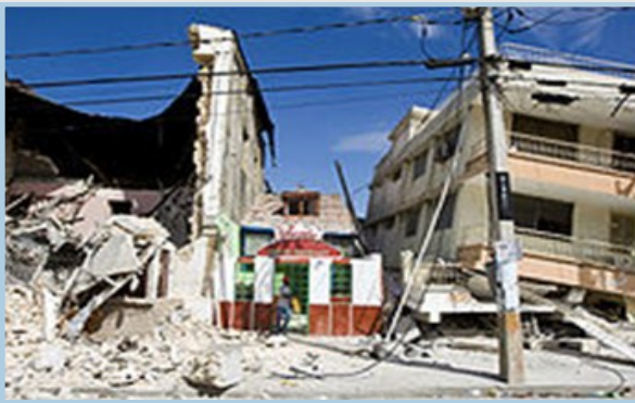
Building damaged in Port-au-Prince
