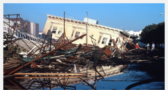
Damage from 2010 Mexicali earthquake
