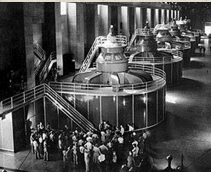
Generators at Boulder Dam supply electrical power to parts of California, Nevada and Arizona.
